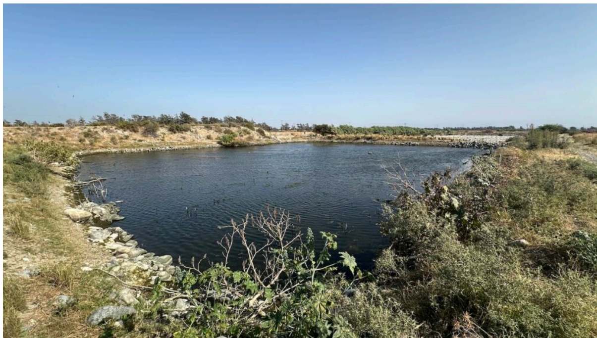
Figure 1. Infiltration pond of the Akrotiri MAR scheme in Cyprus
