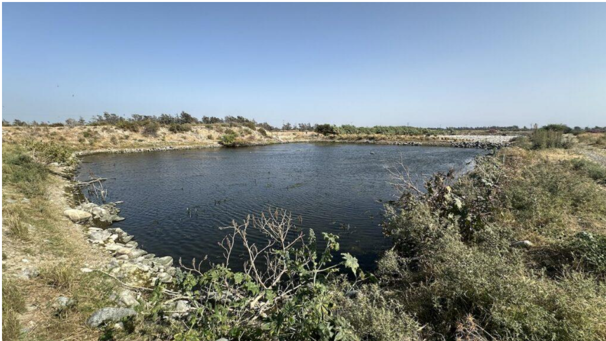
Figure 3. Infiltration pond of the Akrotiri MAR scheme in Cyprus
